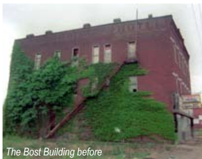
The Bost Building before
